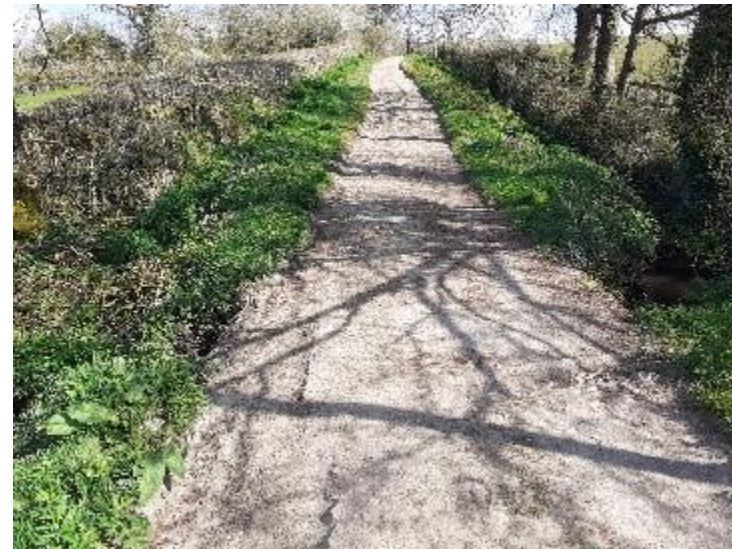
Between B and C, looking north.
